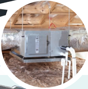
Indoor Fan Coil Unit installed within a roof space
